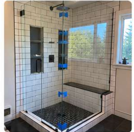
Shower Installed (New Westminster)
