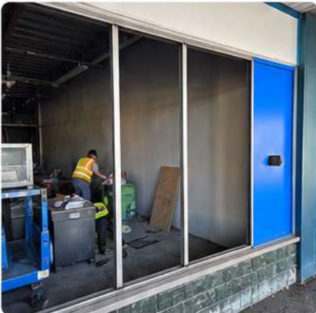
Blue metal panel replaced (Vancouver)
