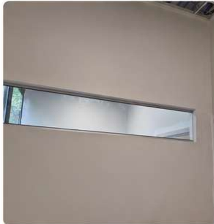
partition Glass Installed (Langley)
